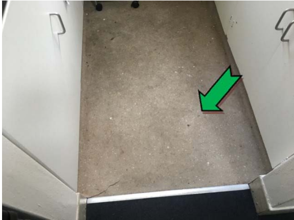
Photo 7. Interior, kitchen, beige floor coverings – non asbestos-containing sheet vinyl.
