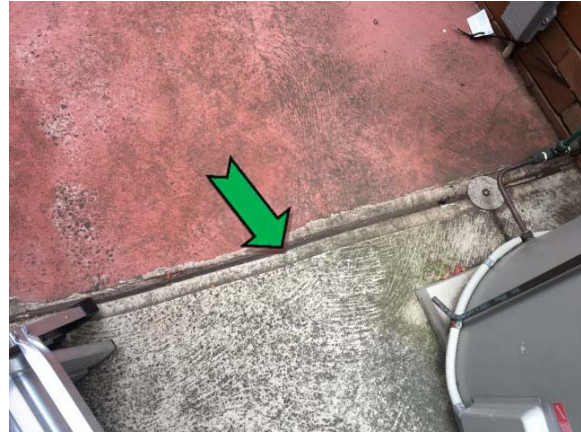
Photo 2. Exterior, north-west elevation, expansion joint – non asbestos-containing construction mastic.
