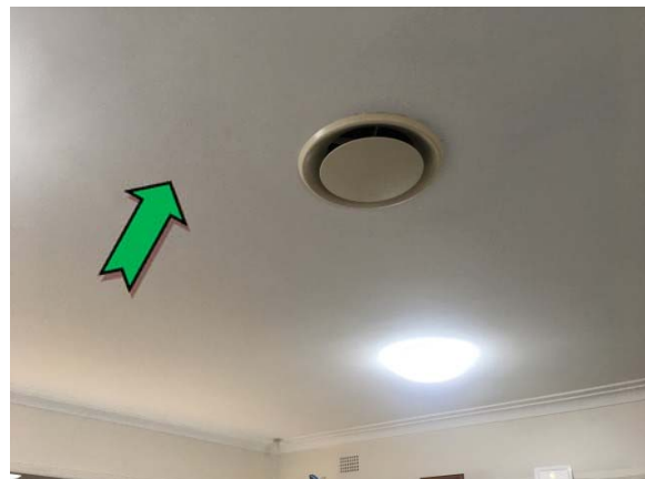
Photo 6. Interior, throughout, ceiling – non asbestos-containing fibre cement sheeting.
