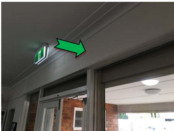
Photo 5. Interior, above entrance, infill panel – non asbestos-containing fibre cement sheeting.
