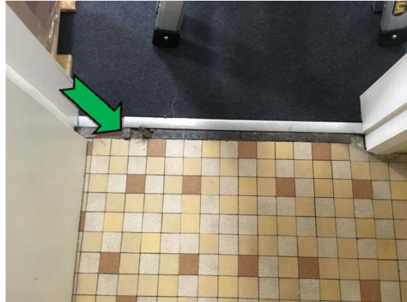
Photo 8. Interior, bathroom, floor coverings, dark grey – non asbestos-containing vinyl floor tiles.
