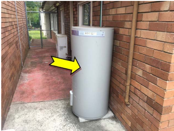
Photo 9. Exterior, north elevation, hot water heater – suspected SMF internal insulation material.
